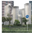
1963 Ventilation Towers Umeda, Kita-ku, Osaka
