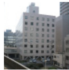
1969 Office Building 16 Ishigatsujicho, Tennoji-ku, Osaka
